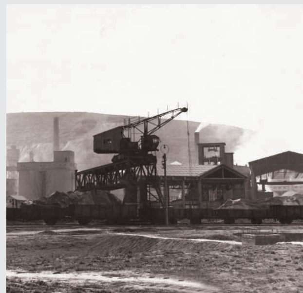
Kran na izgrađenom depou uglja troske i gipsa / Crane on the built coal, slag and gypsum open storage
